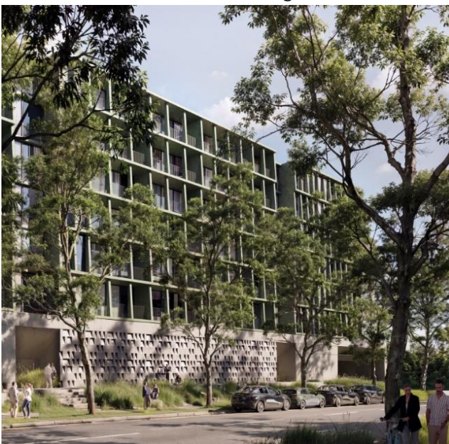
View of the Young Street frontage
